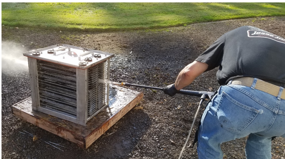
Figure 3-8-1 ESP Cell "Cautious Pressure Washing"
