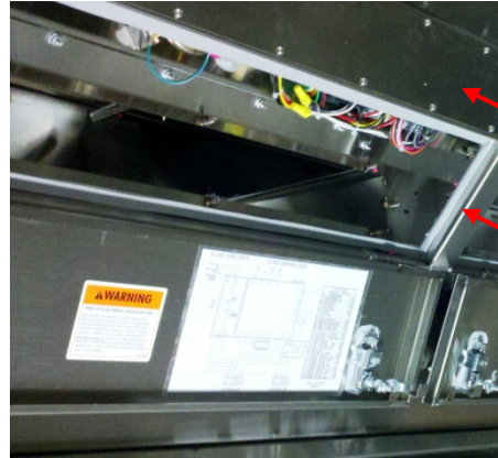
Figure 6-31-1 Main Electrical Raceway Access Panel
