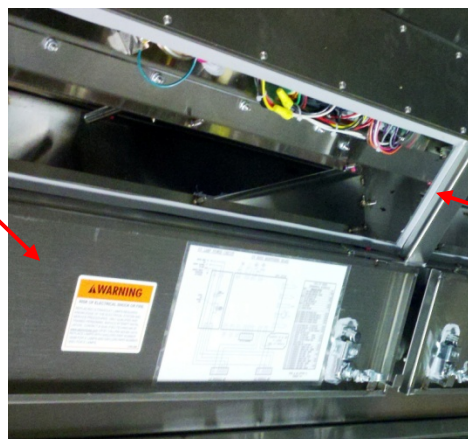
Figure 4-5-3 UV Module Access Door
