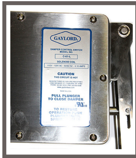
A. 12671 – C-61-L DAMPER CONTROL SWITCH
